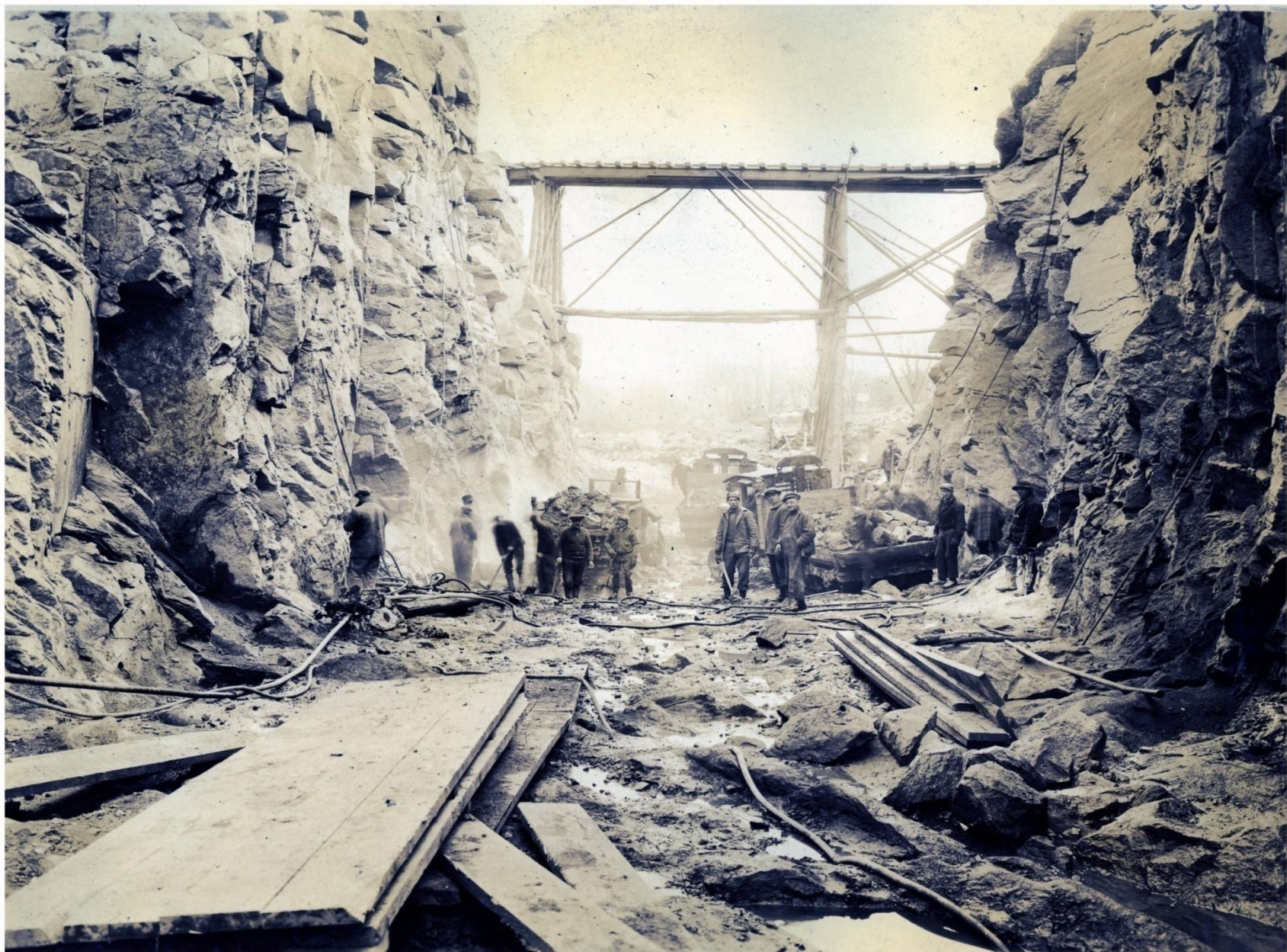
View of outlet channel.
