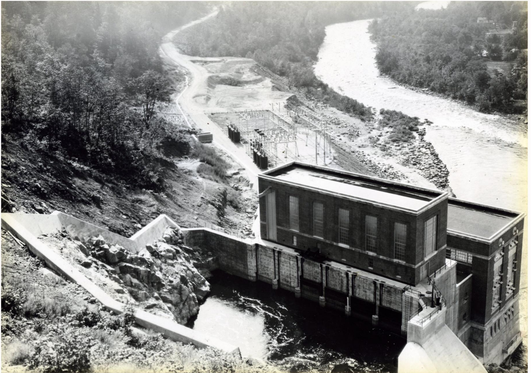
View of Fore Bay at Power House. Transformer and switching station in middle background.
