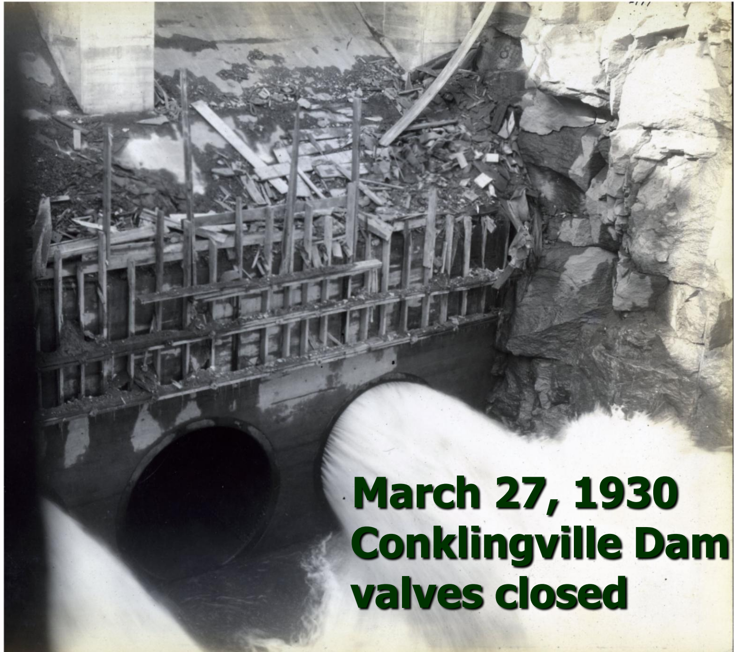
View showing outlet with one valve closed.
