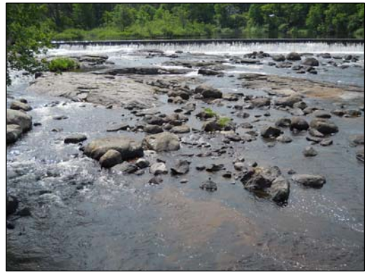
Photo 3 – Ledge outcropping downstream of the Hawkinsville Dam.
