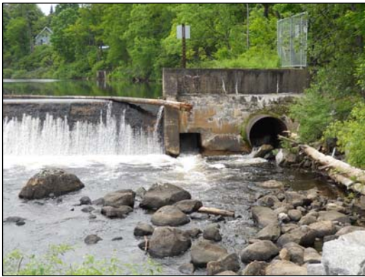
Photo 2 – Low-level impoundment drain and penstock on river-left bank.
