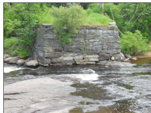
Photo 4 – Historic bridge abutment downstream of the Hawkinsville Dam, river-right bank.
