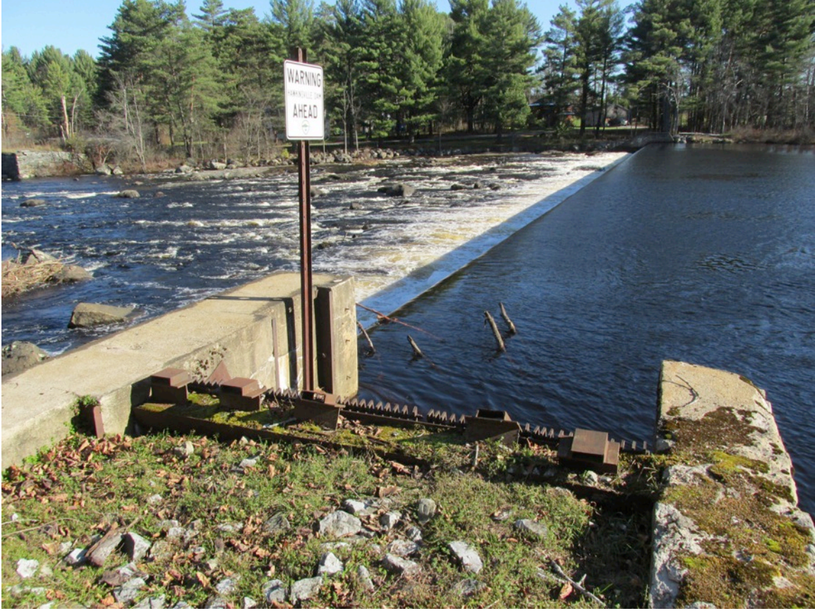
Figure 7. Dam and intake looking NE, 2013.
