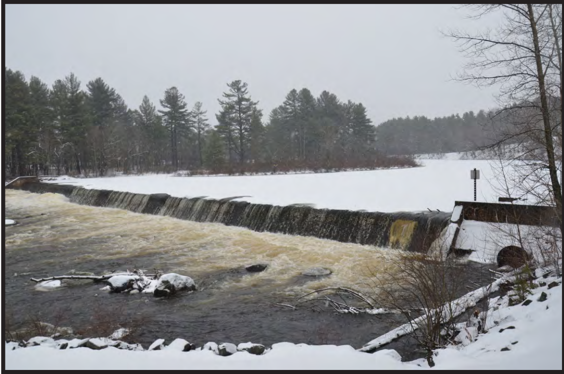
Photograph 1: Hawkinsville Dam, View to Southeast
