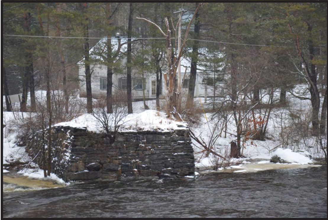
Photograph 2: Historic Bridge Abutment, View to East
