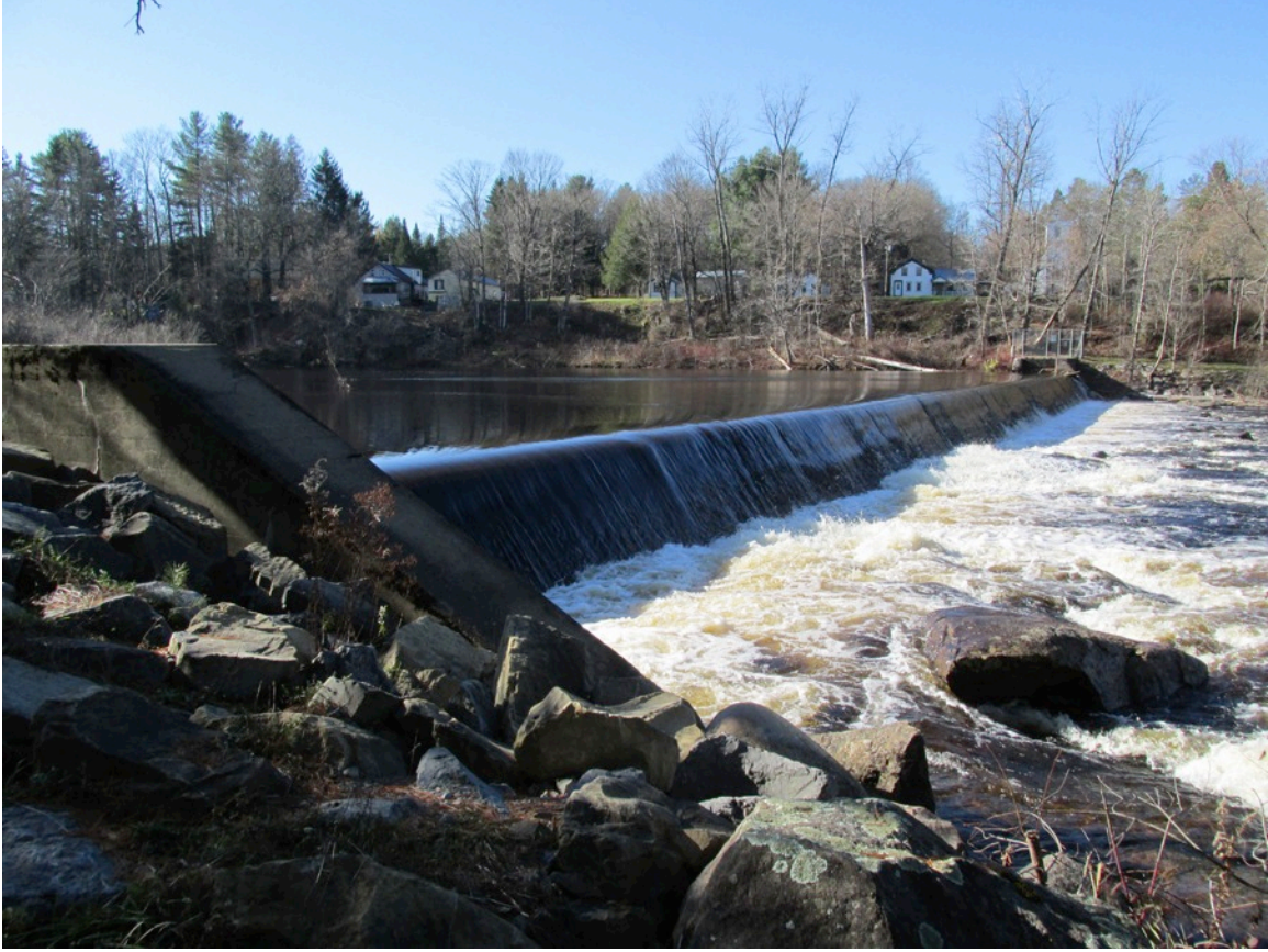
Figure 9. Downstream face of dam looking SW, 2013.
