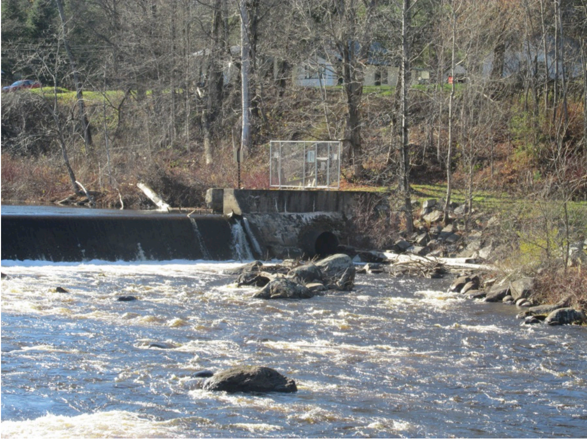
Figure 11. Downstream face of intake, showing penstock outlet.
