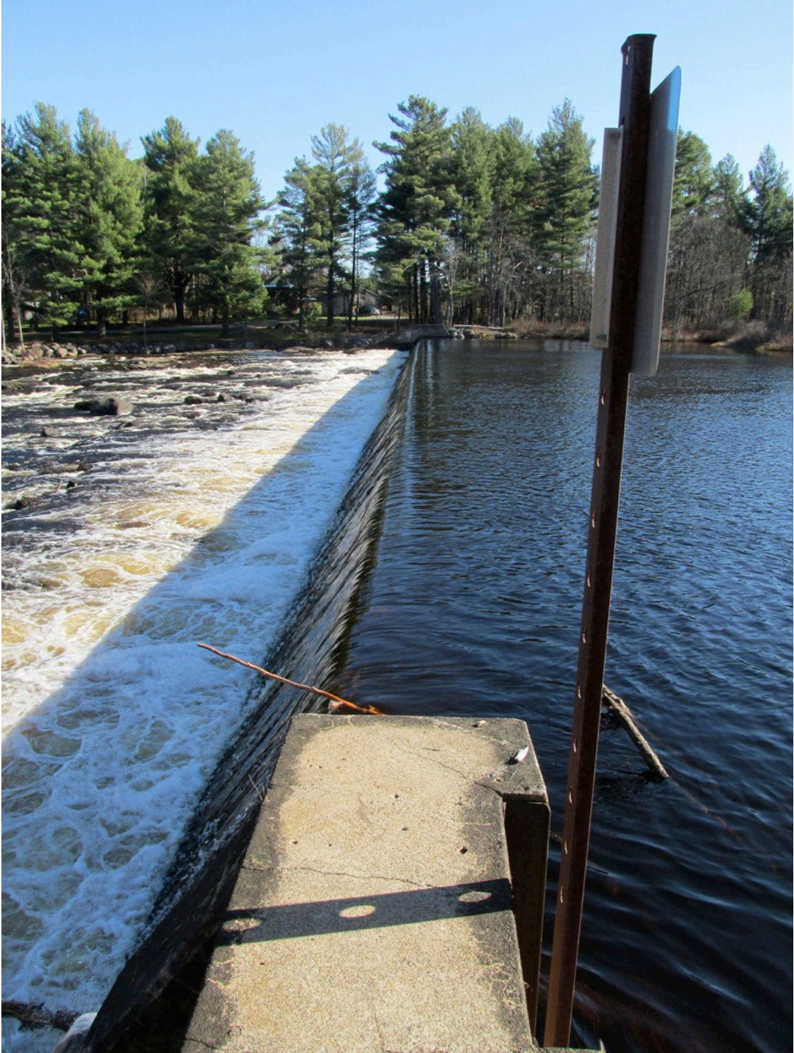
Figure 6. Crest of dam looking E, 2013.
