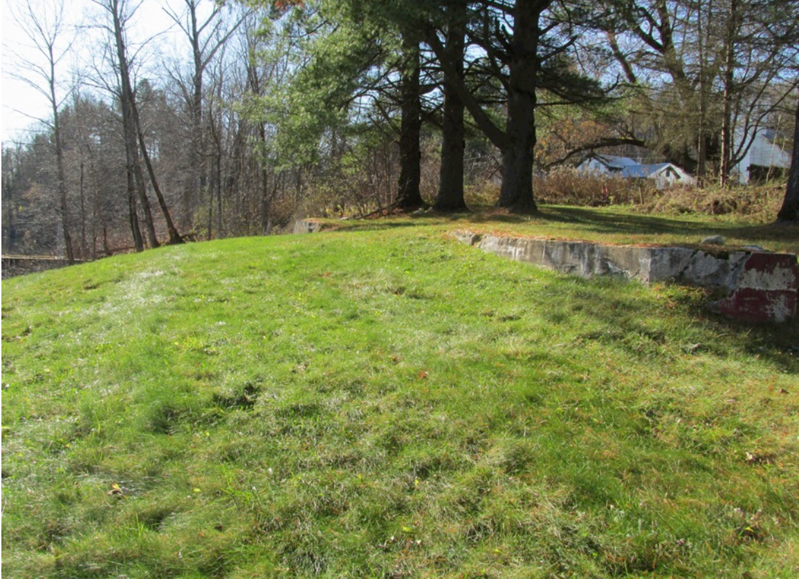
Figure 13. Former factory site, foundation detail, 2013.
