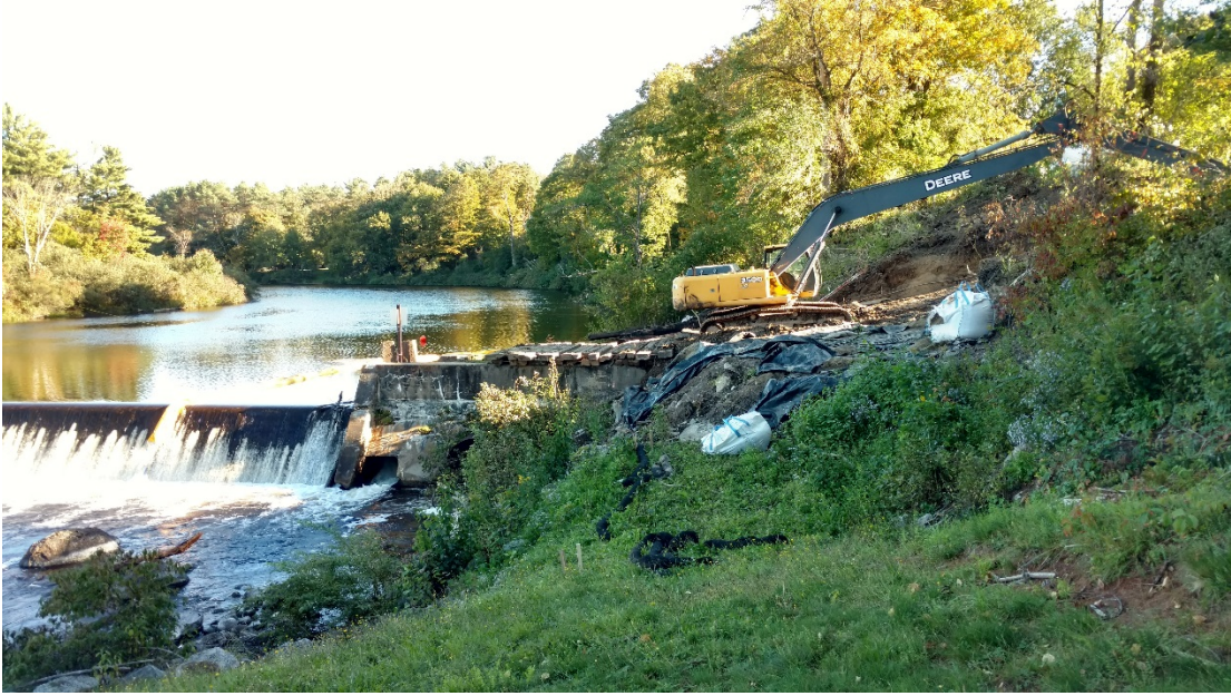
West side access preparation
