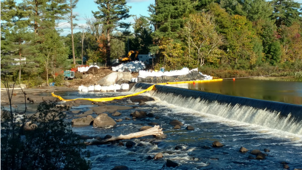
East side coffer dam and turbidity curtain installed
