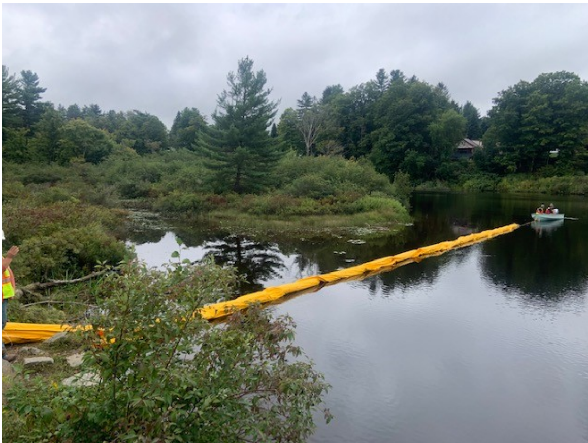
Turbidity Curtain Installation – east side
