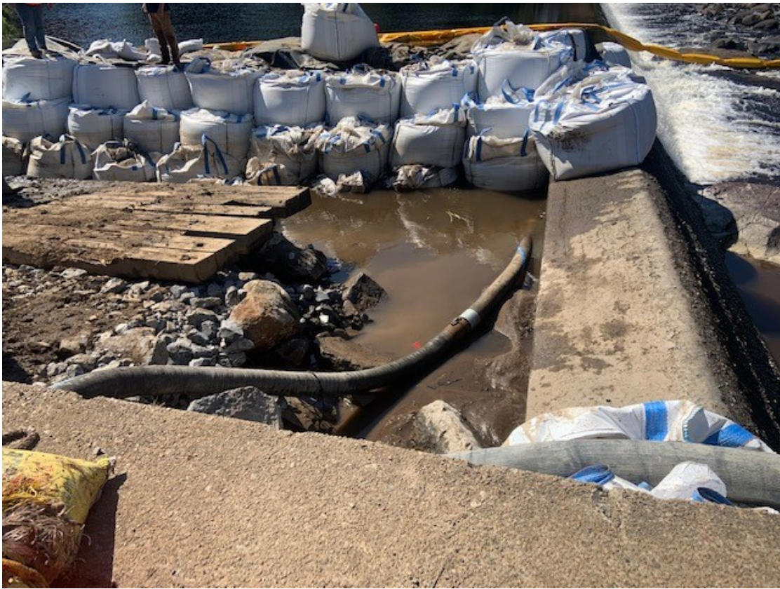
Dewatering east abutment
