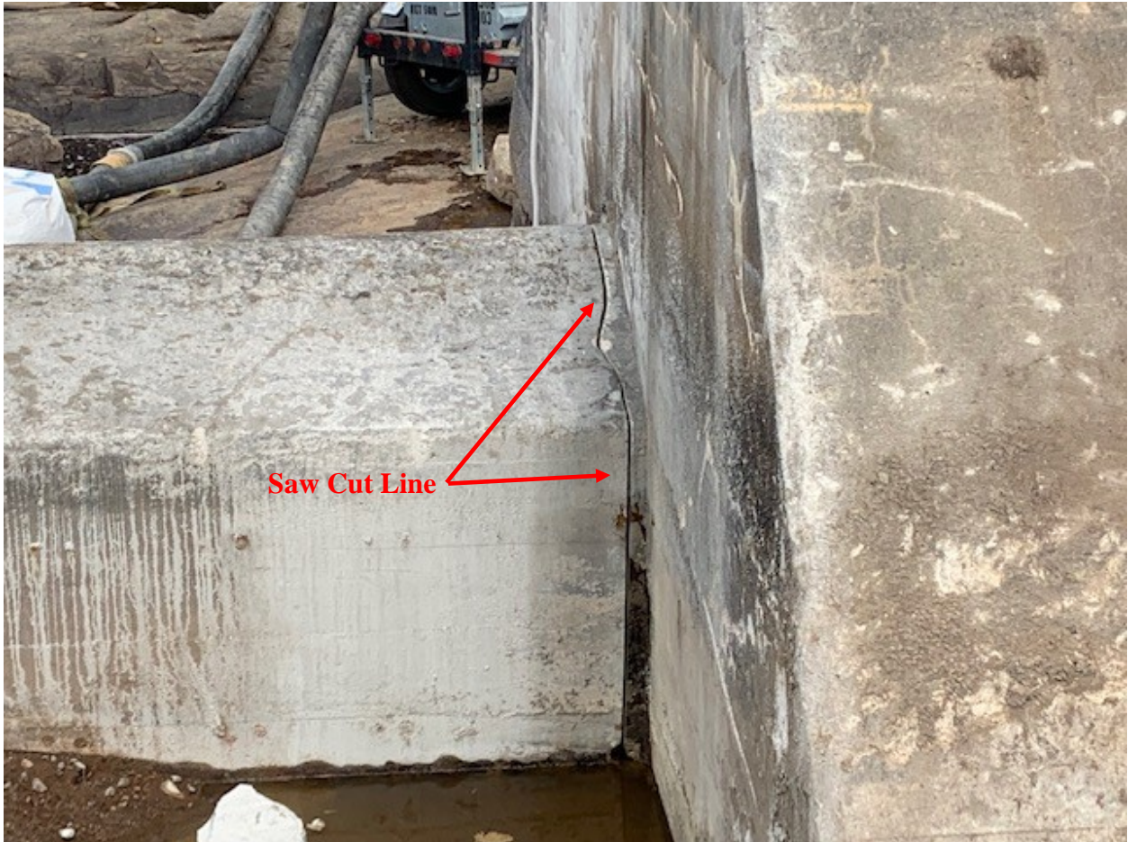
Saw cut at east end of spillway
