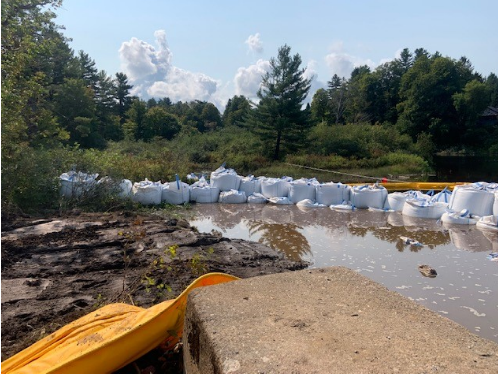
Sand bag cofferdam installation – east side
