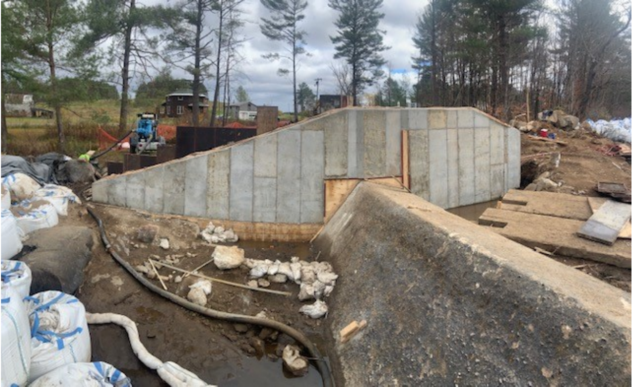
Completed concrete abutment at east-side (view east)
