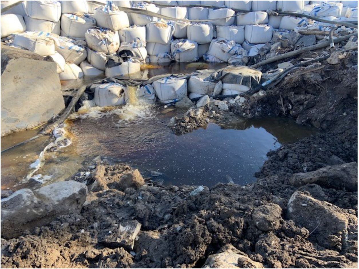
Sand bag cofferdam upstream of west end of spillway (view south-east)
