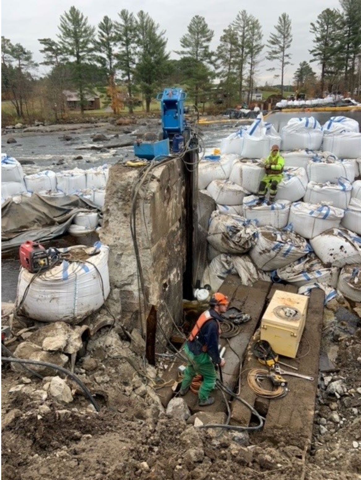
Saw cutting of west end of spillway (view south)
