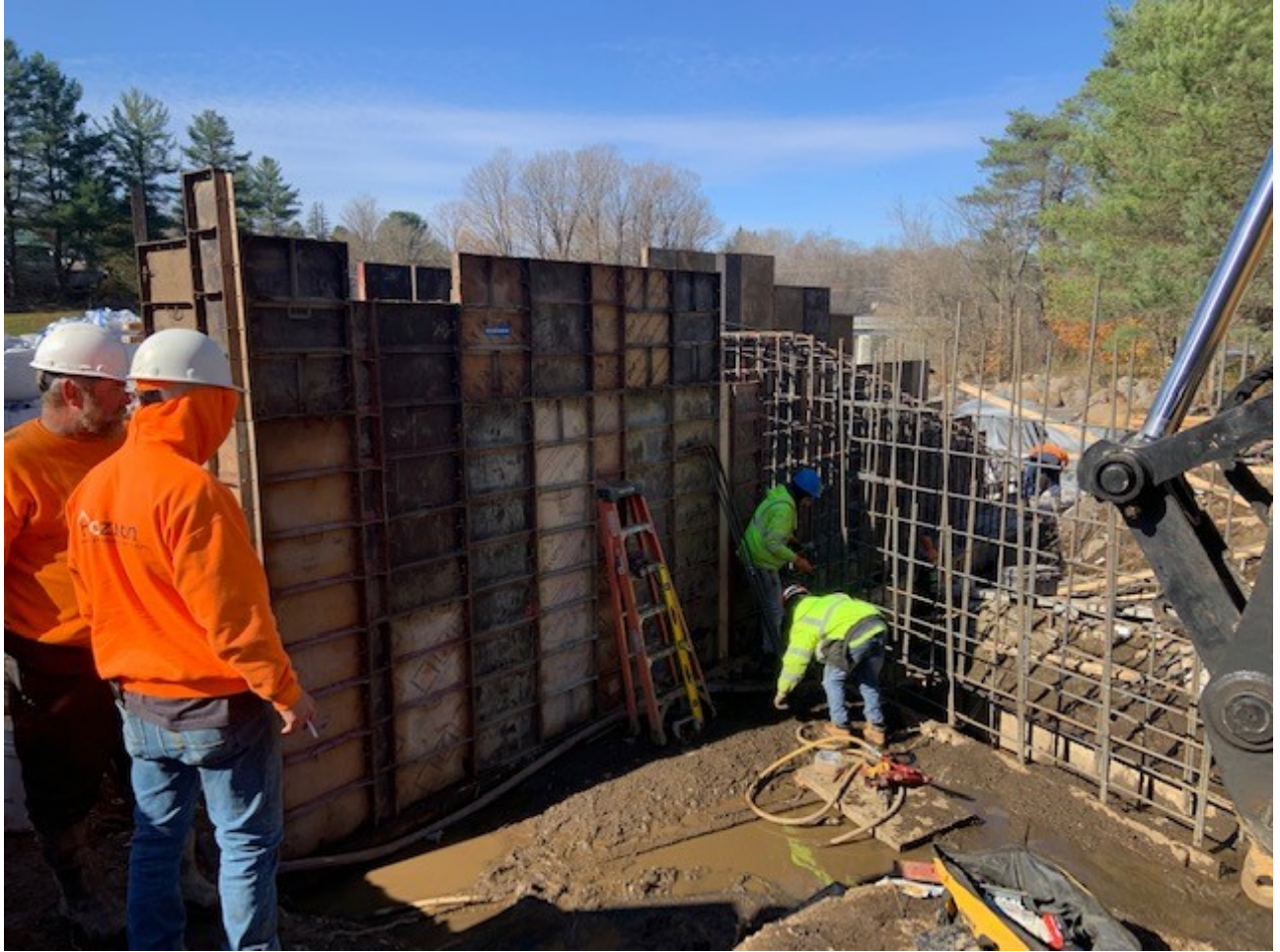
Concrete forms for abutment and reinforcing steel for cut-off wall at east-side (view north-west)
