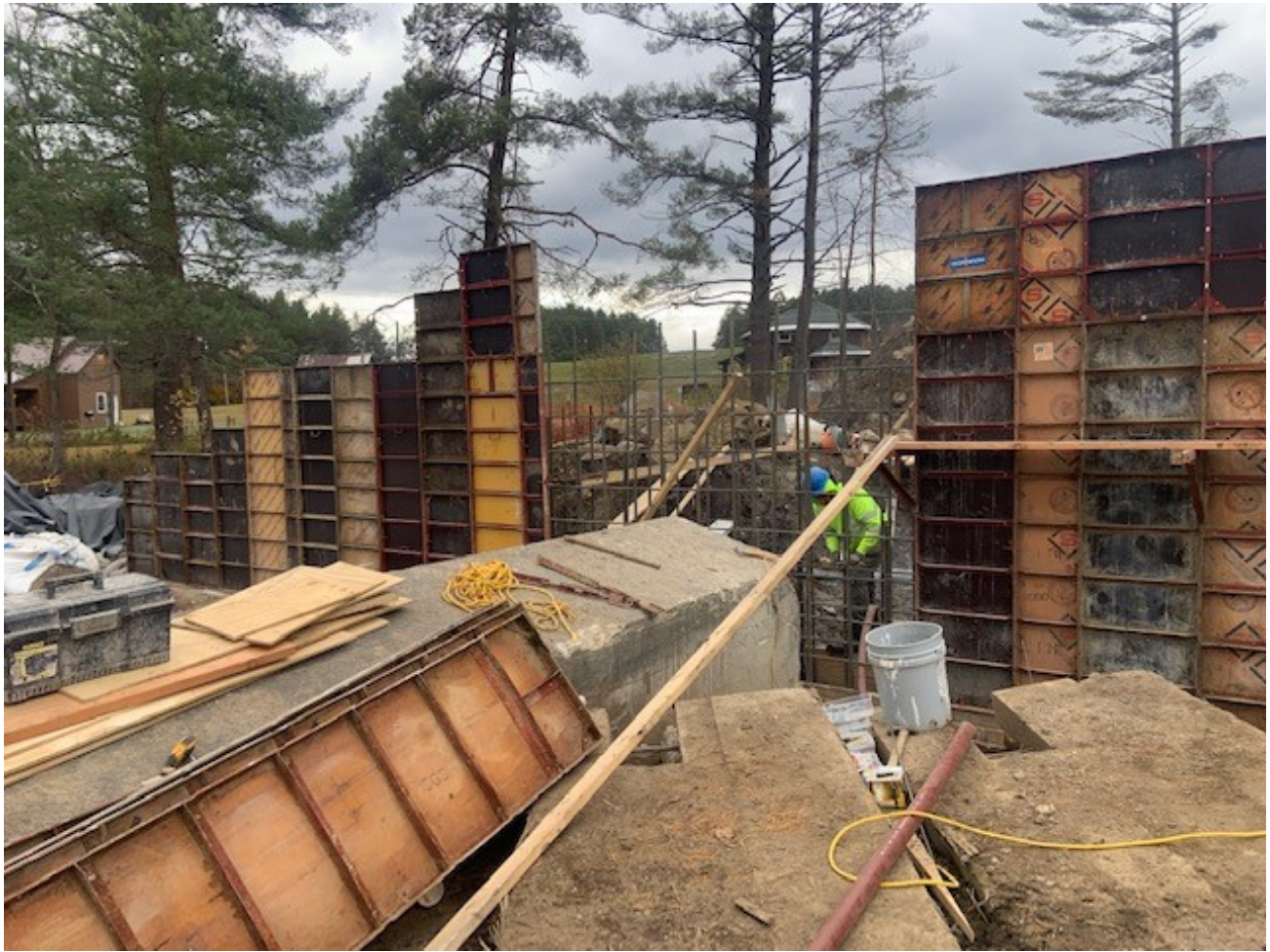
Concrete forms and reinforcing steel at east-side abutment (view east)
