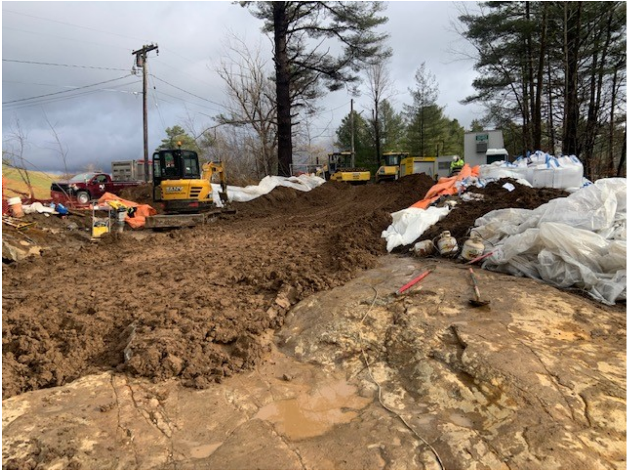
Start of placement of embankment core material (view south-east)
