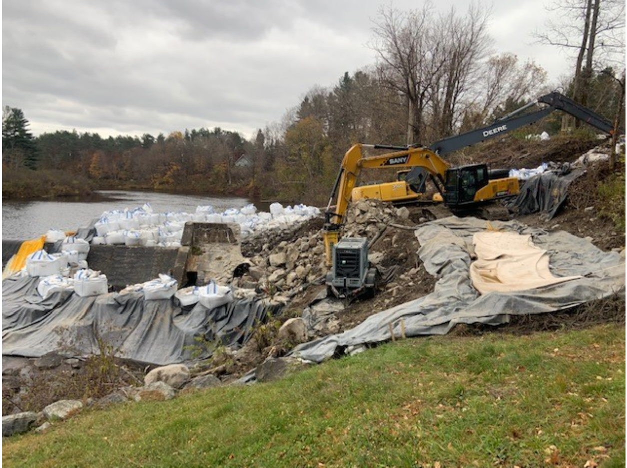
Start of west-side outlet structure concrete demolition and excavation of exiting bank fill (view south)
