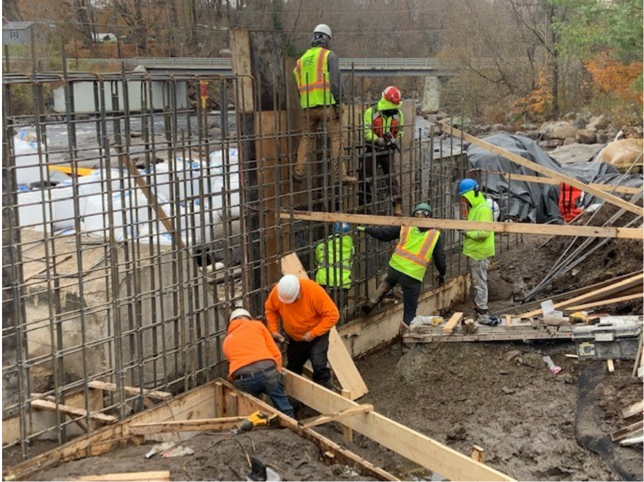
Reinforcing steel at east-side abutment and start of concrete form construction for cutoff wall (view north-west)
