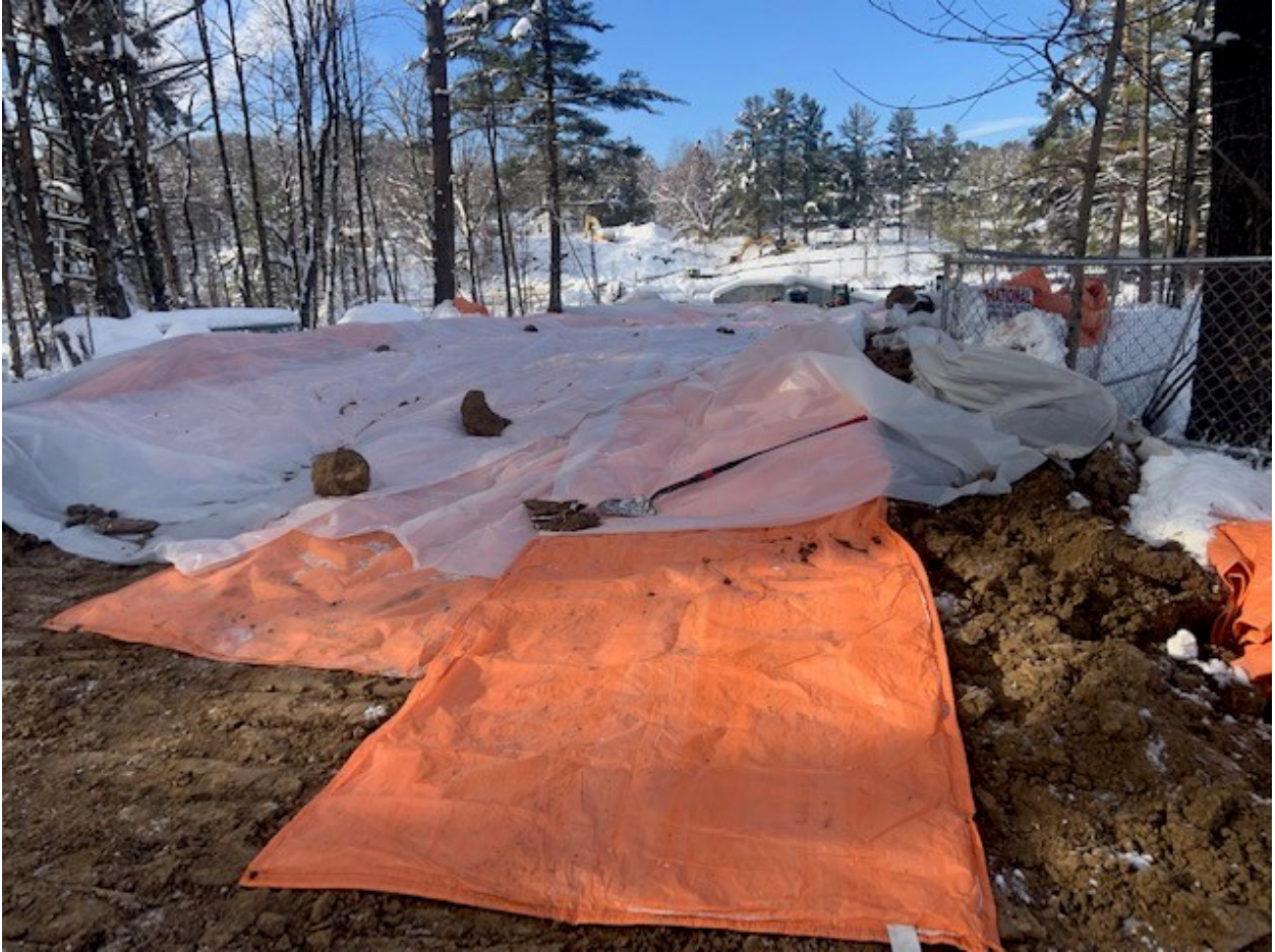
Winter weather protection of embankment core material (view west)
