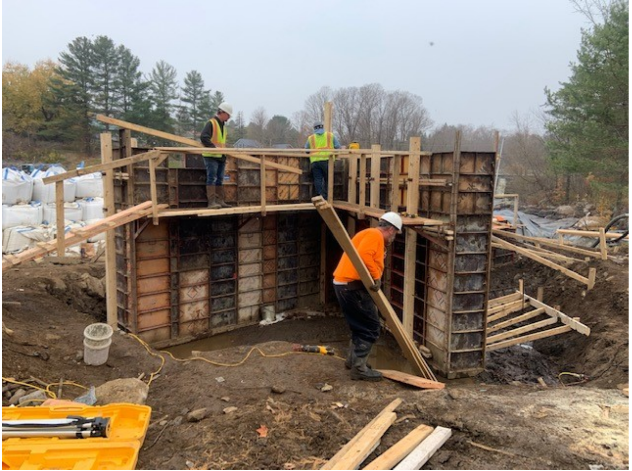
Concrete forms for abutment and cut-off wall at east-side (view north-west)
