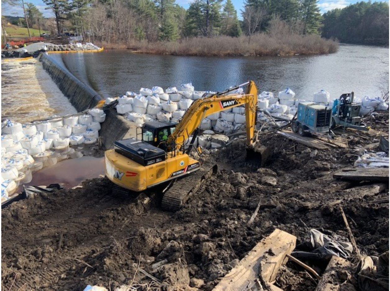
Excavation at west end of spillway (view south-east)
