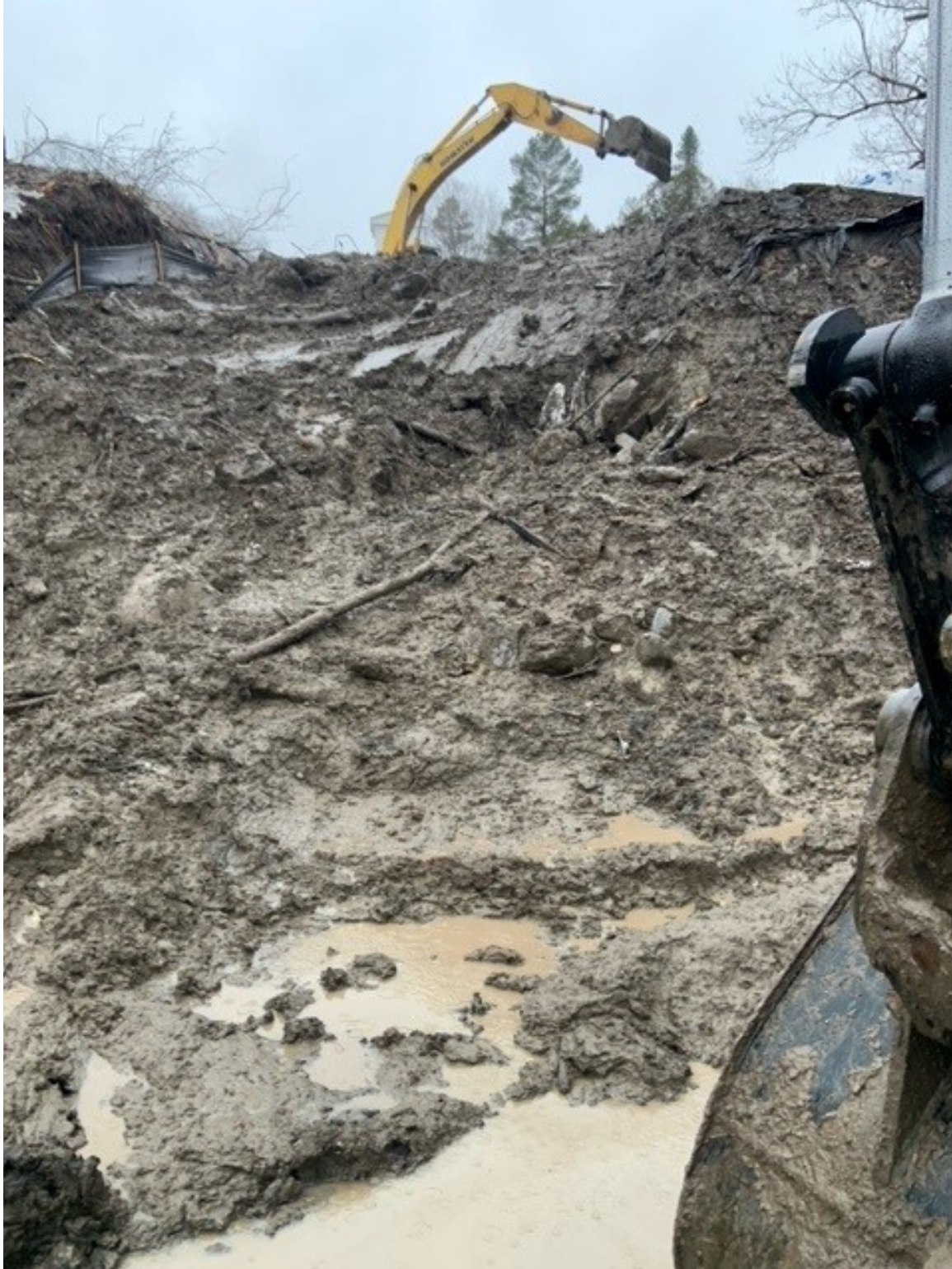
Excavation at west-side bank (view west)
