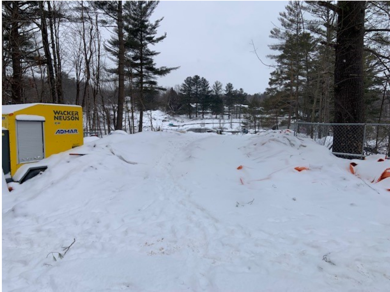
Winter weather protection of embankment core material under 12 inches of snow on December 27, 2022 (view west)
