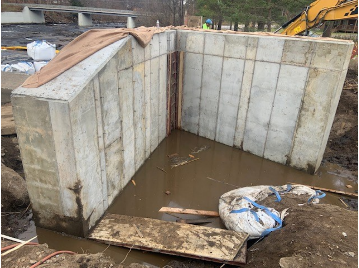
Completed concrete abutment and cut-off wall at east-side (view north)
