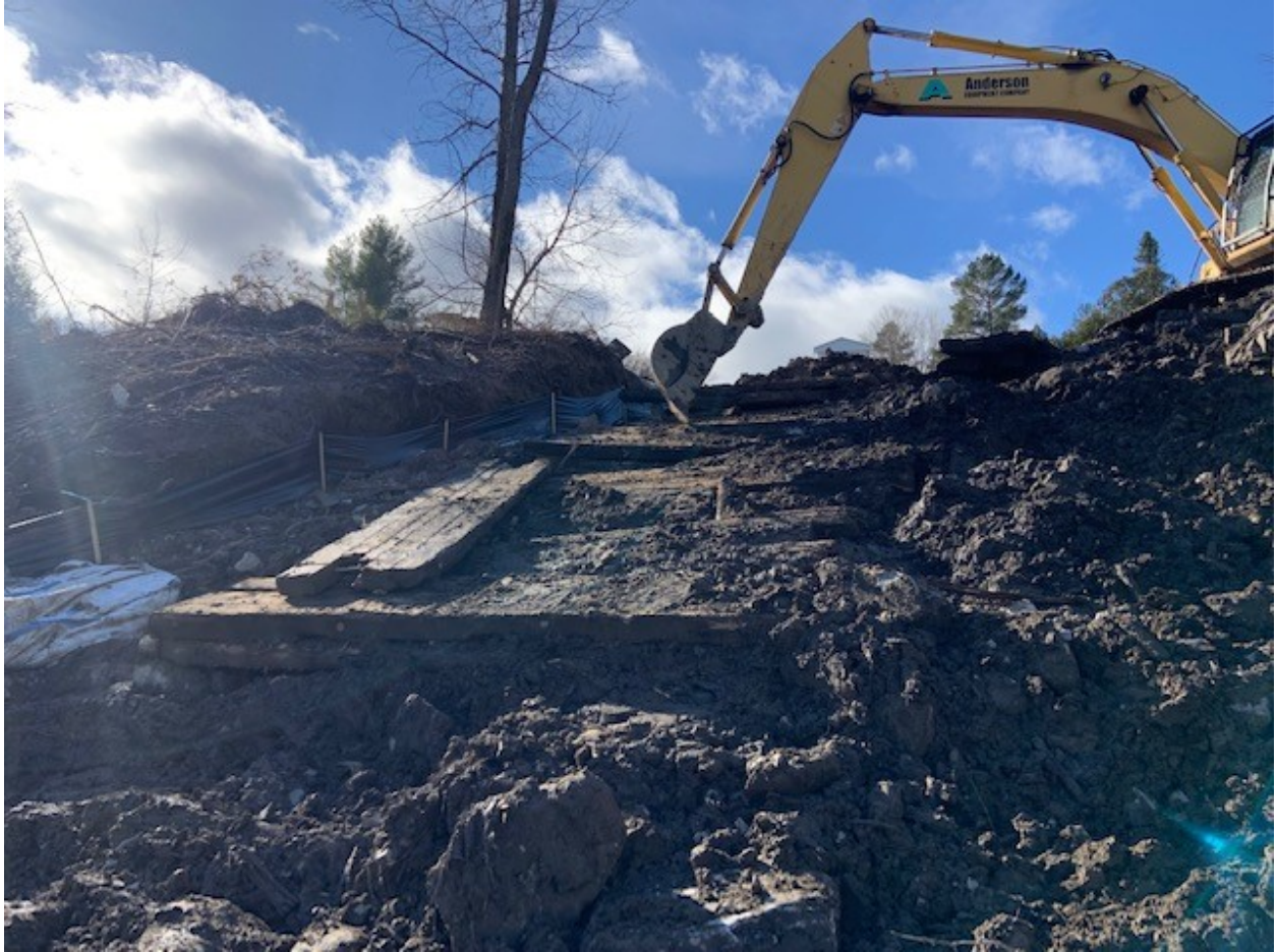
Excavation at west-side bank (view south-west)
