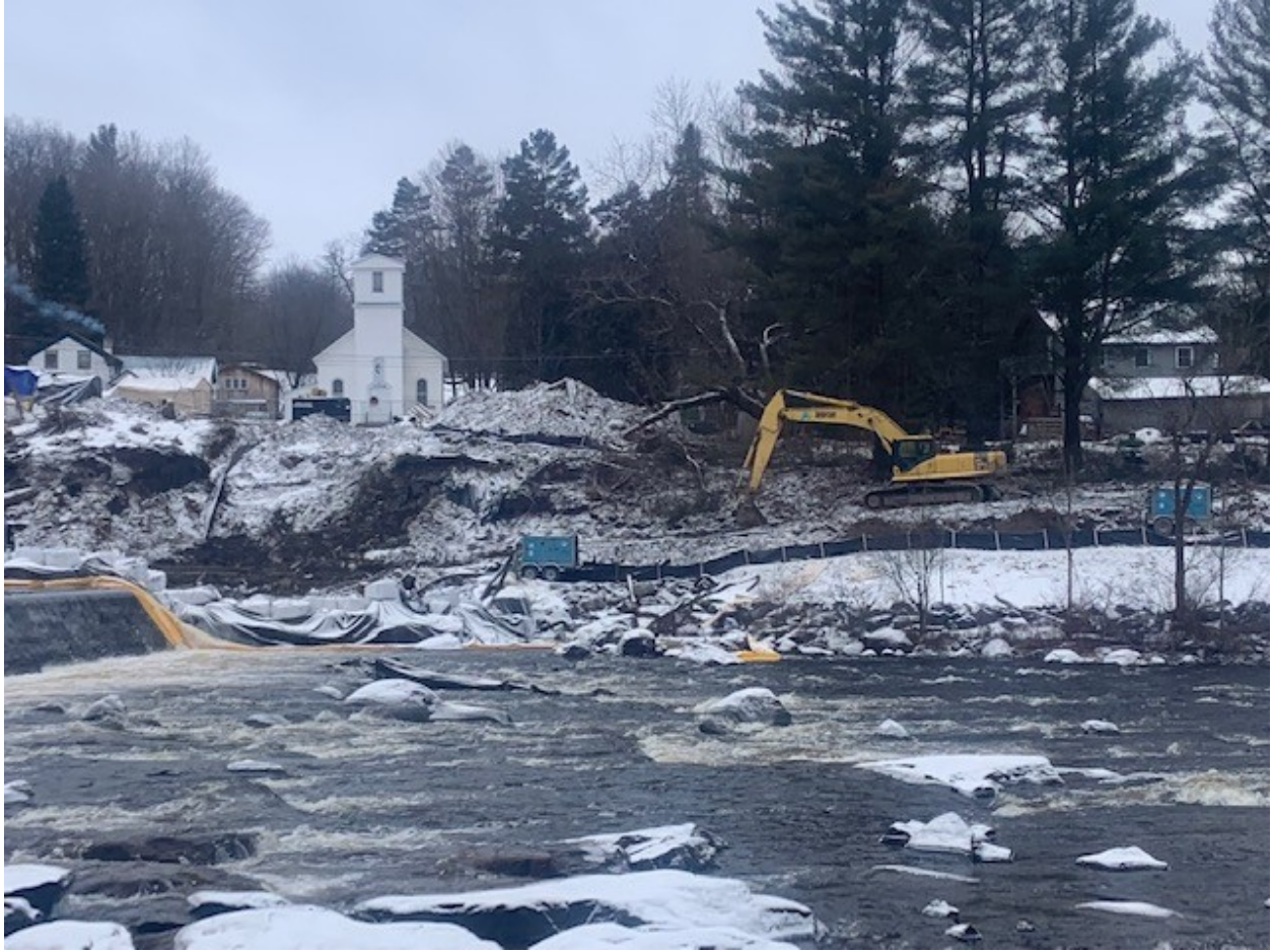
West bank - access road construction (view to west; loose soils area left side of photo)
