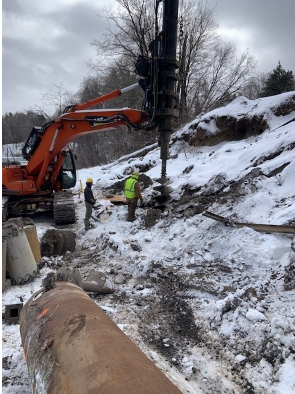
Drill for temporary pile and shoring wall installation
