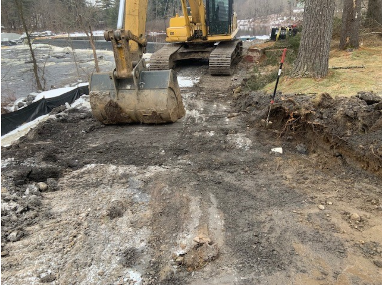
Construction of west side access road (view upstream, spillway - top of photo in background)
