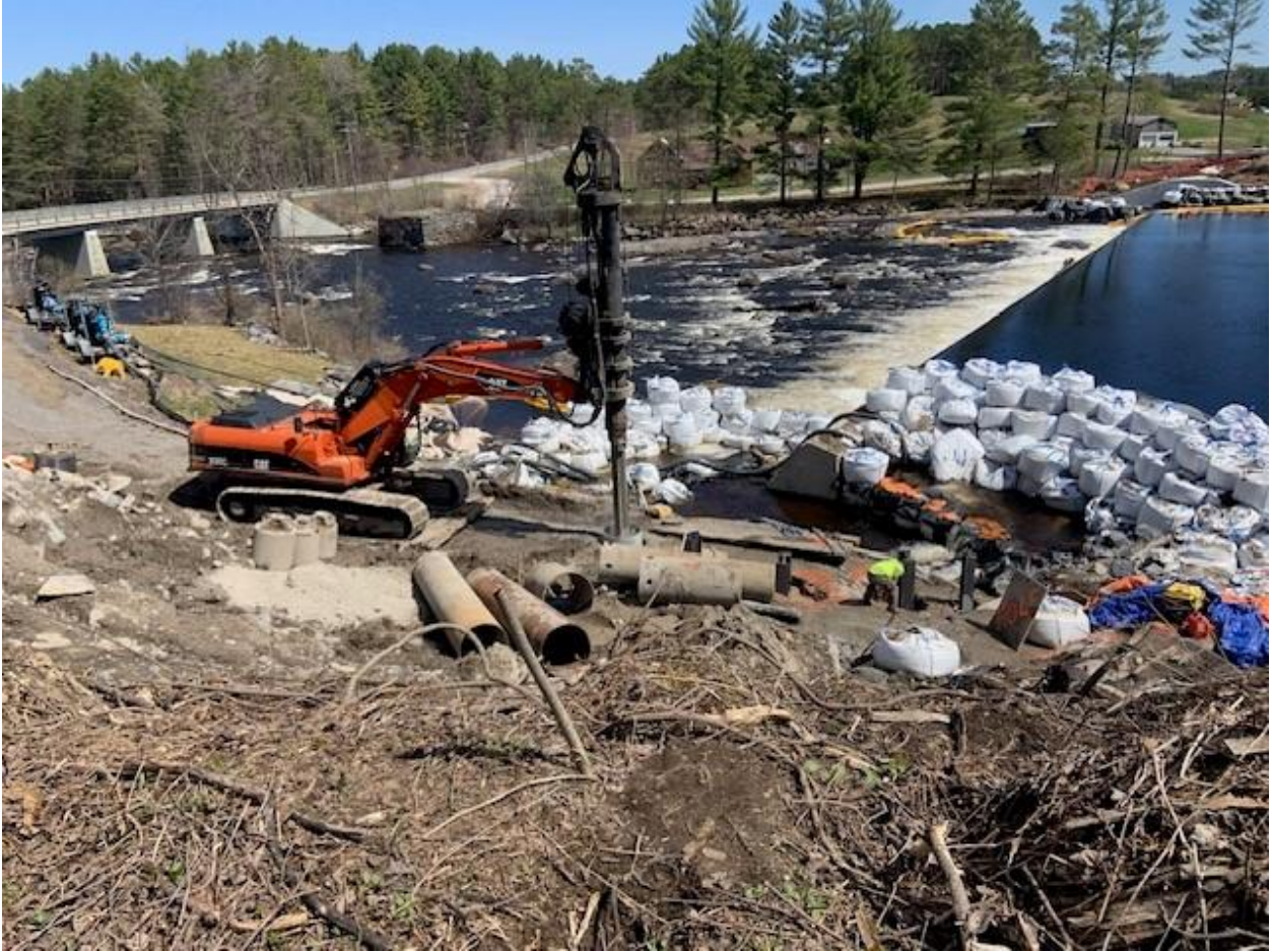
Additional pile construction
