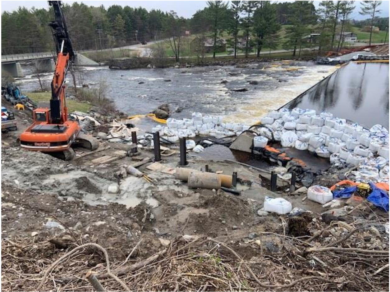
Installed piles for shoring system
