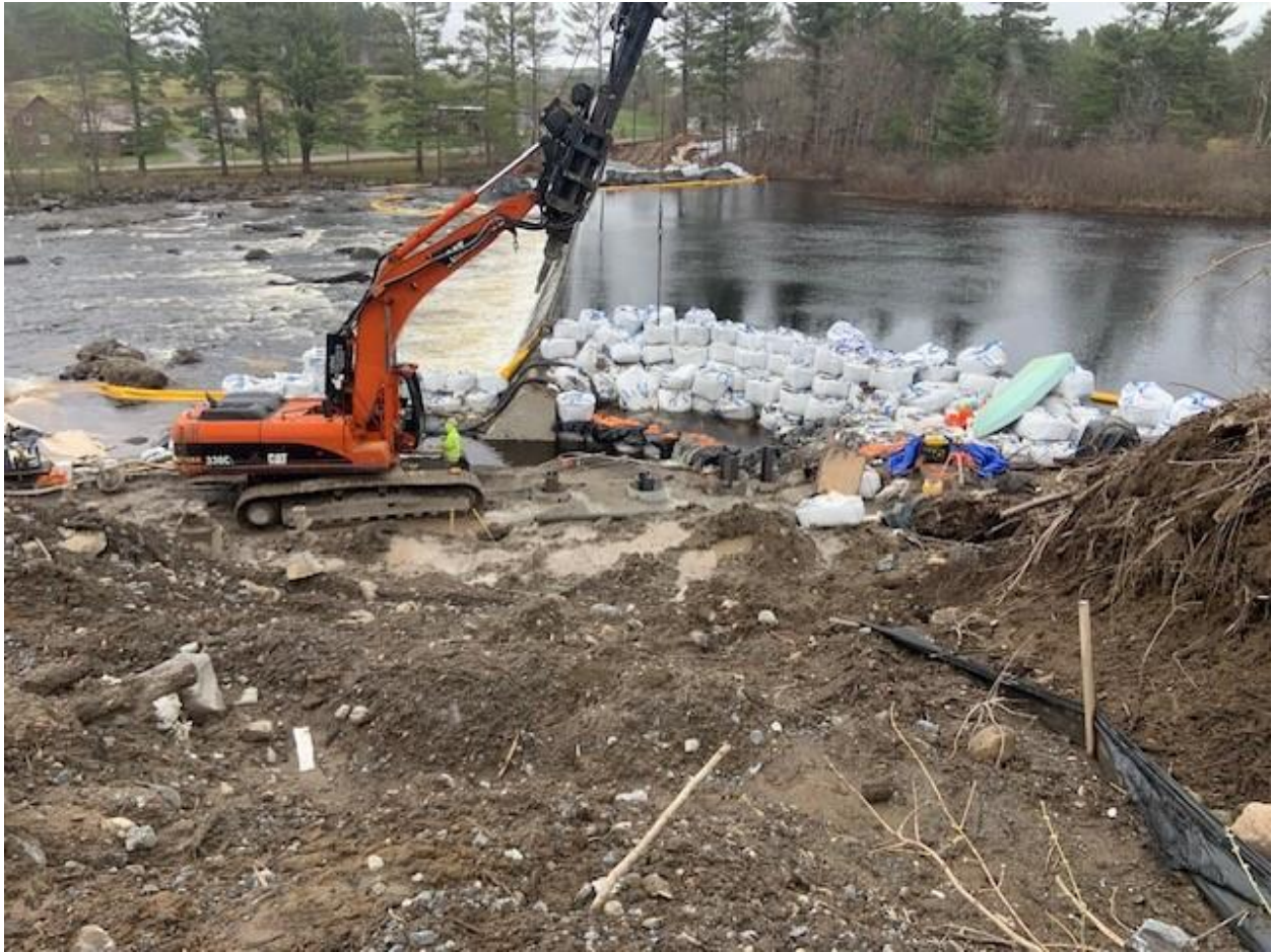
Rock drilling and installation of steel piles for west bank shoring system
