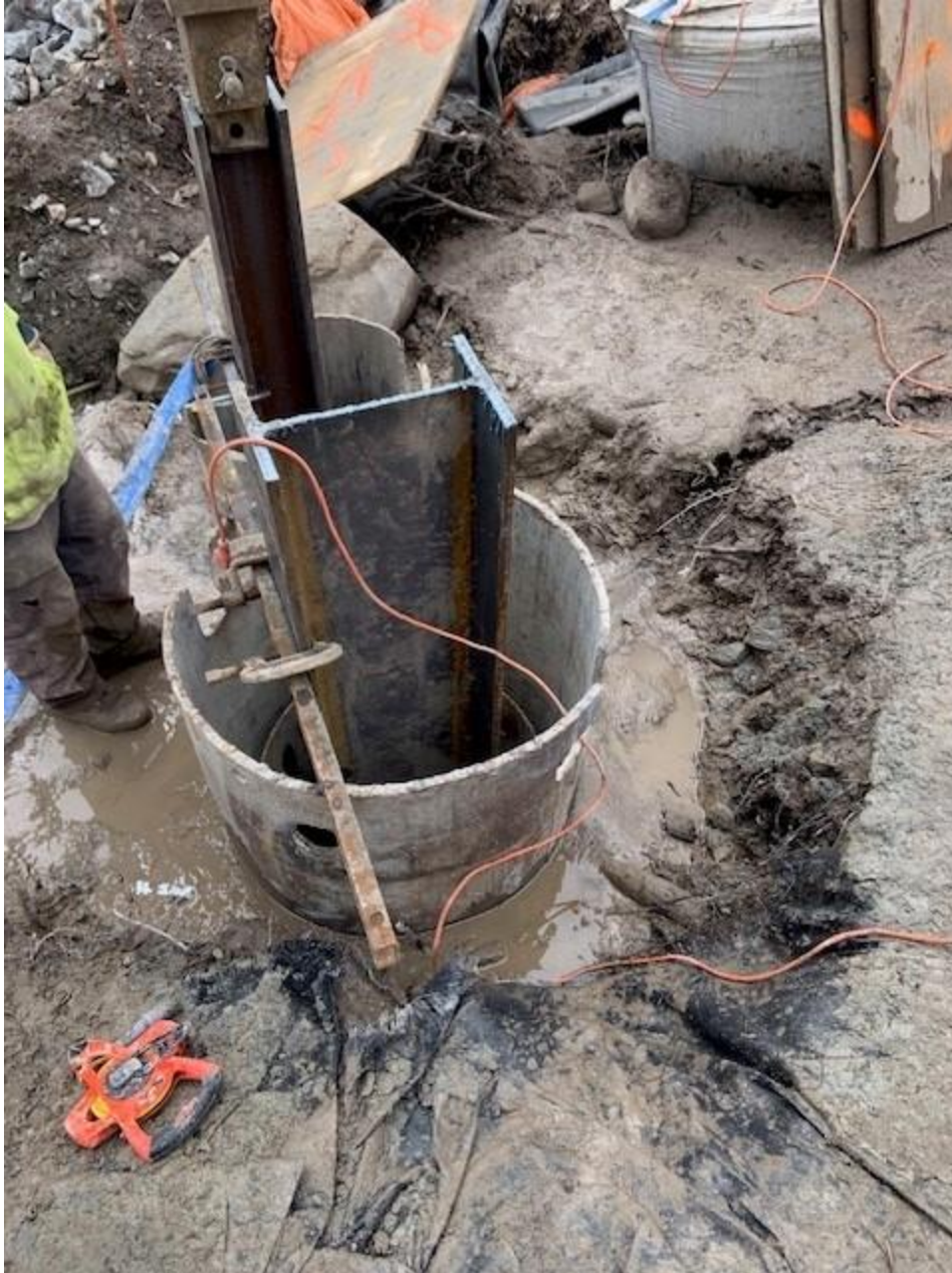
Steel pile in casing prepared for concrete placement
