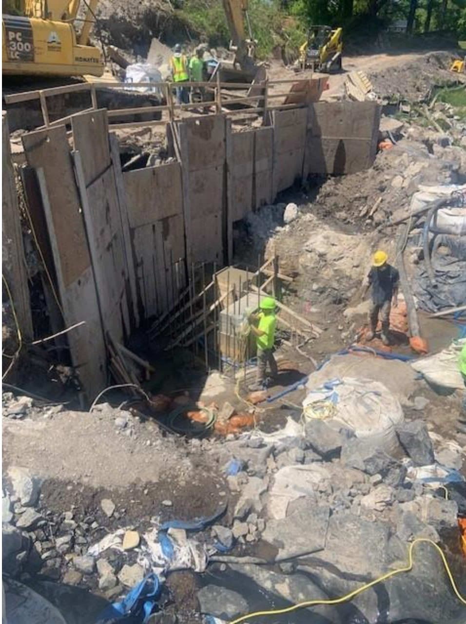
Outlet pipe saddles - cured concrete form removal.
