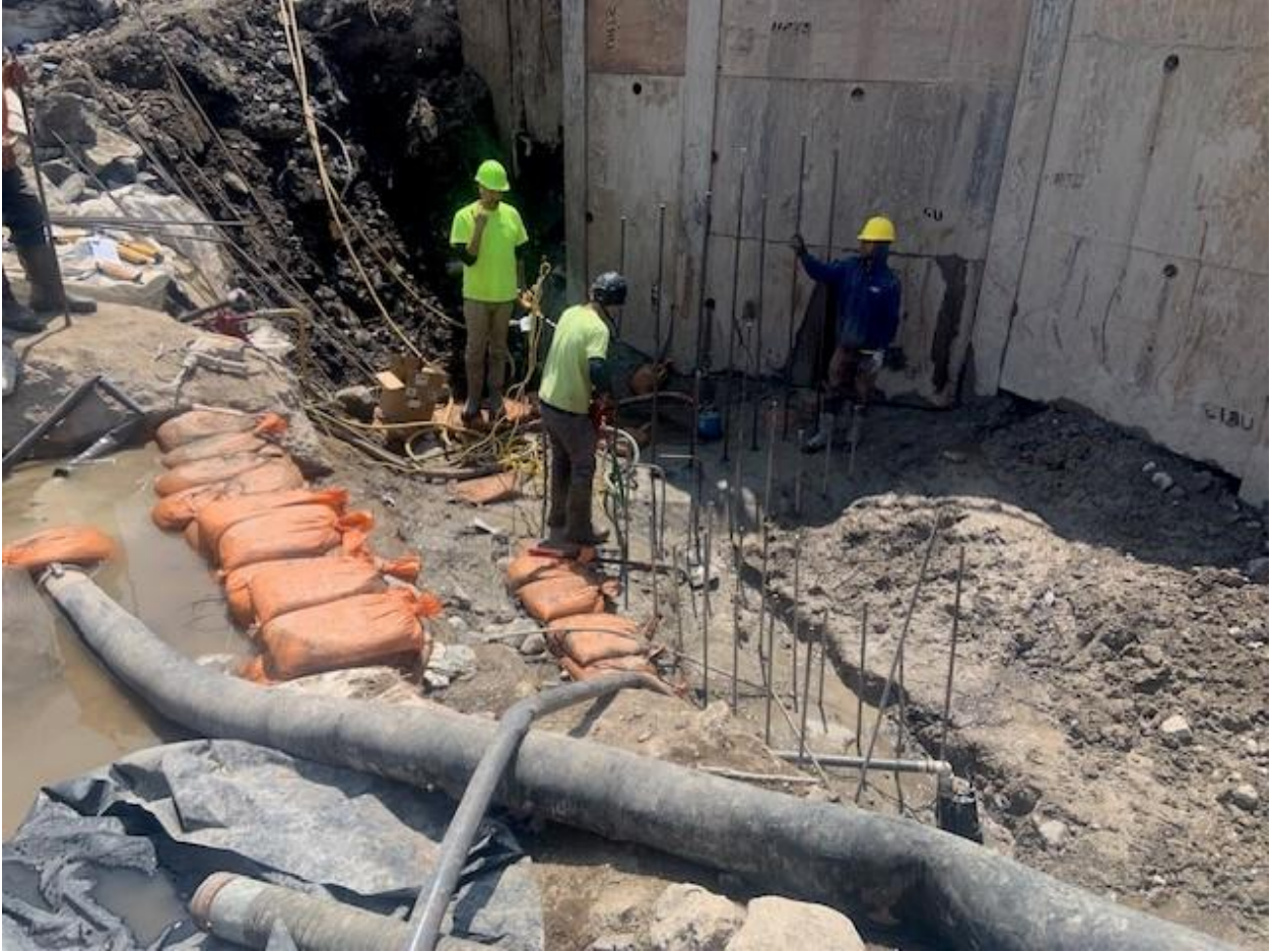
Installation of rock dowels.
