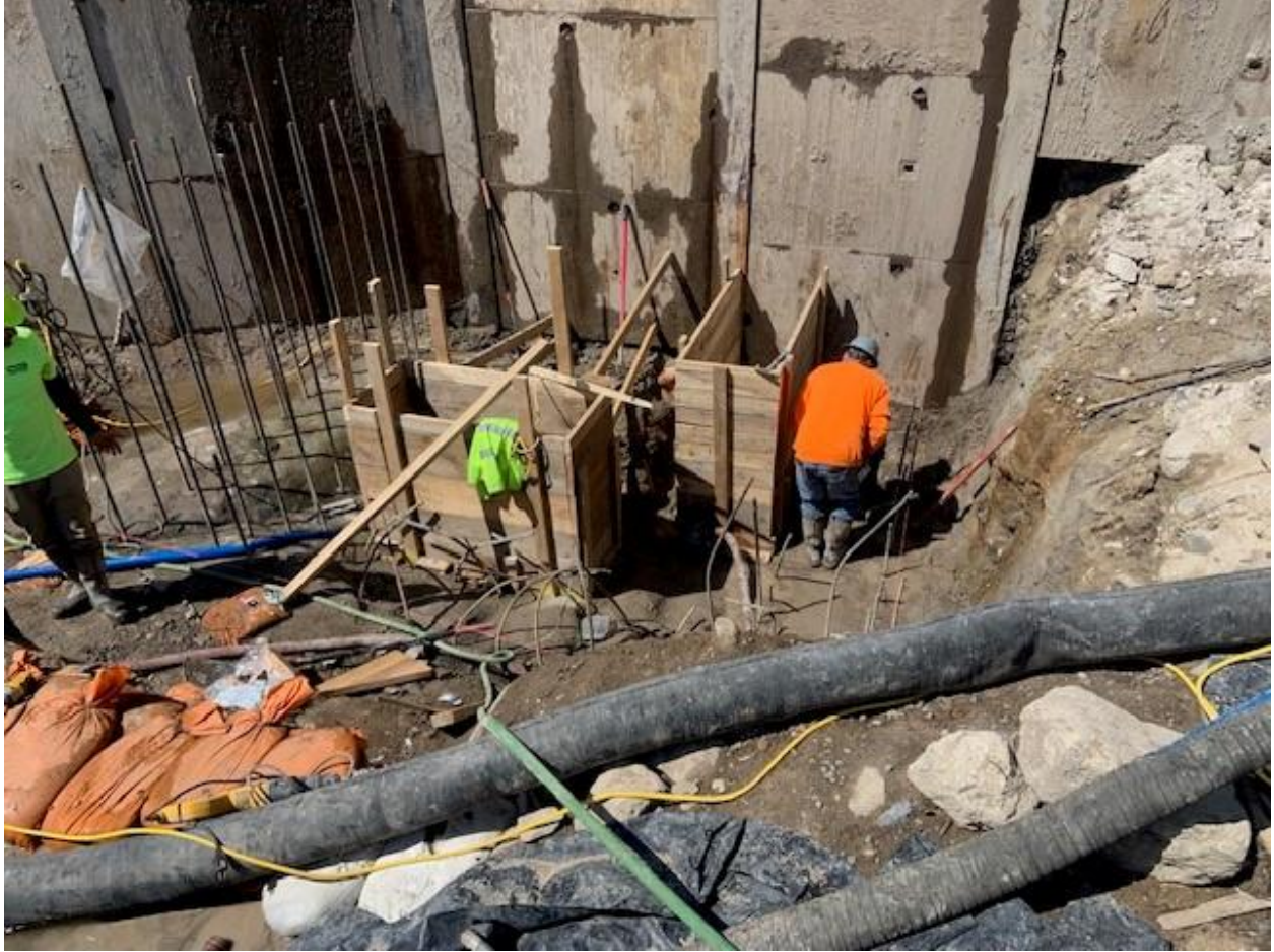
Concrete forms for outlet pipe saddles.
