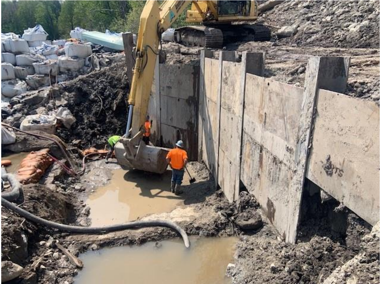
Installation of the west bank shoring system and excavation.
