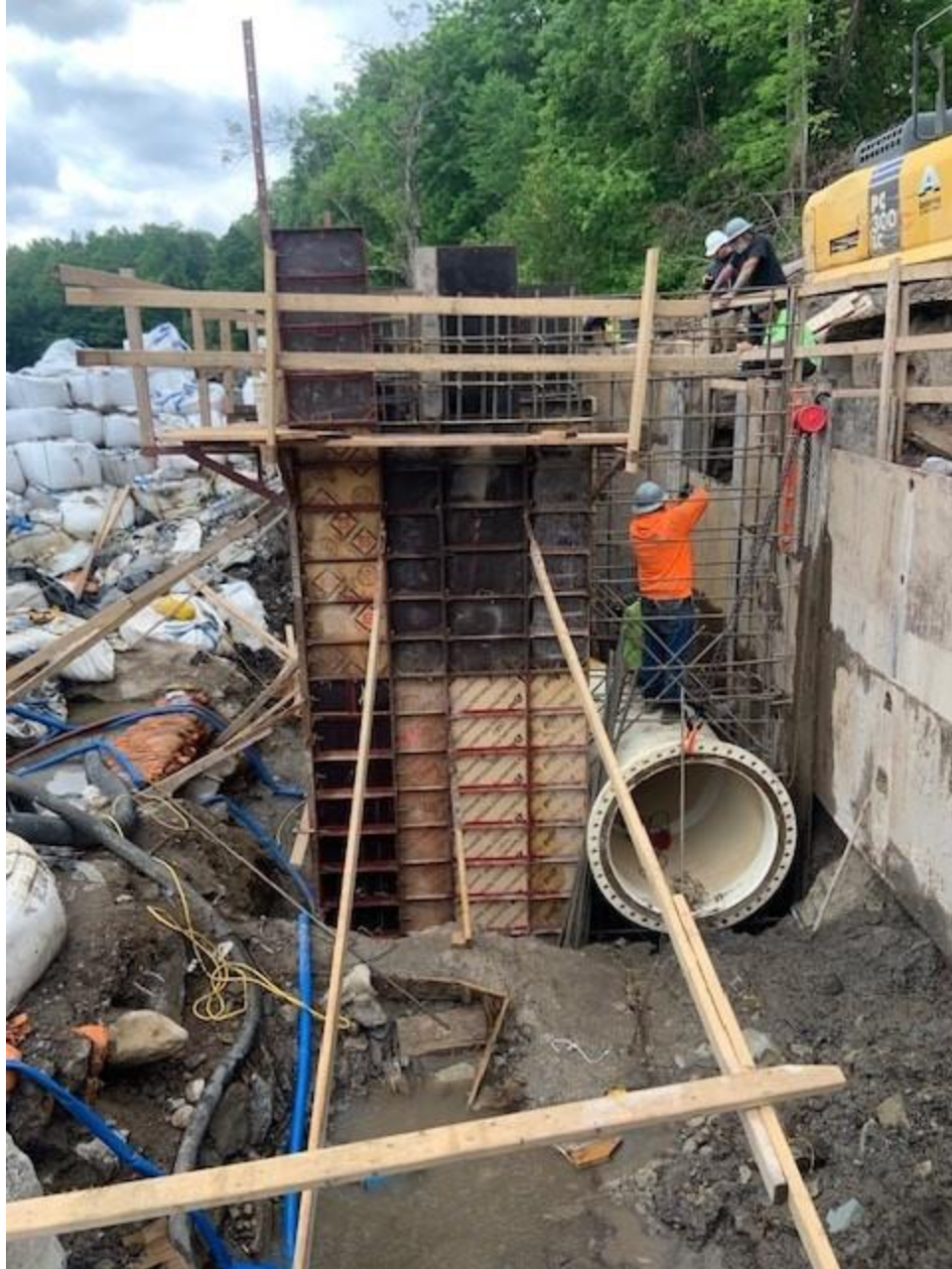
Steel reinforcement and formwork for concrete abutment wall and cut-off wall.
