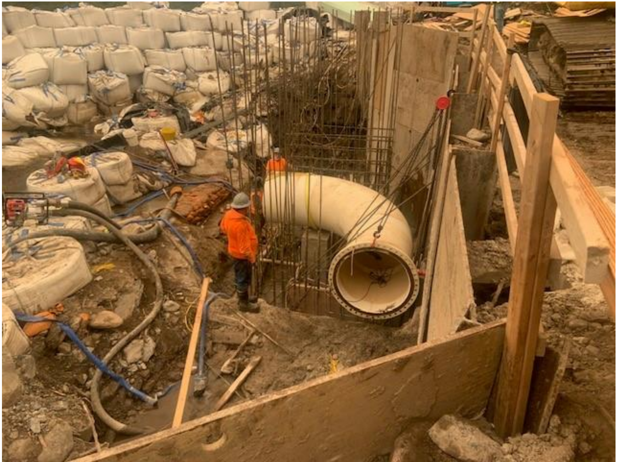
Installation of embankment dam core material (east side).
