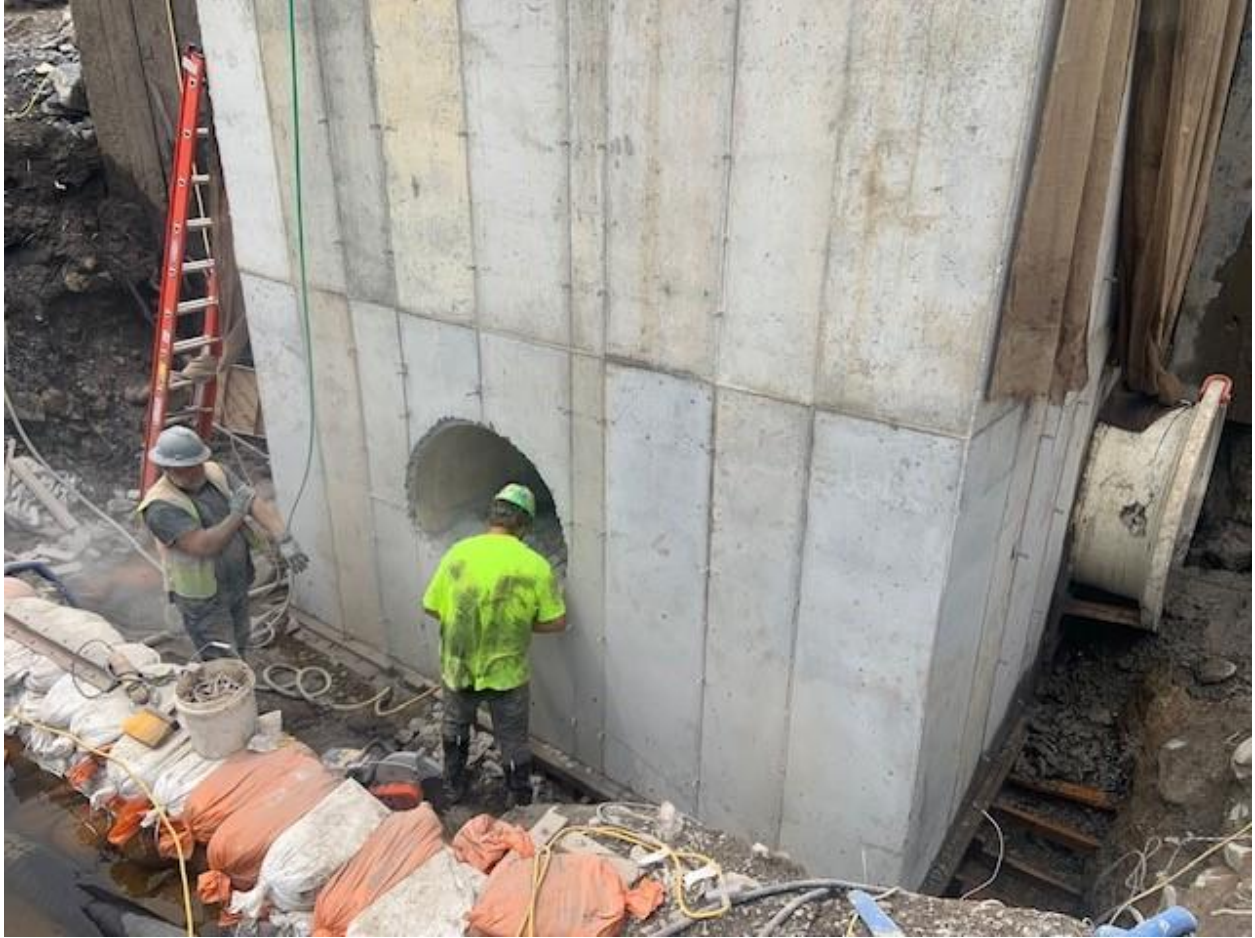
Concrete abutment at intake-side of outlet pipe (foreground) and pipe flange connection at cut-off wall (right side of photo).
