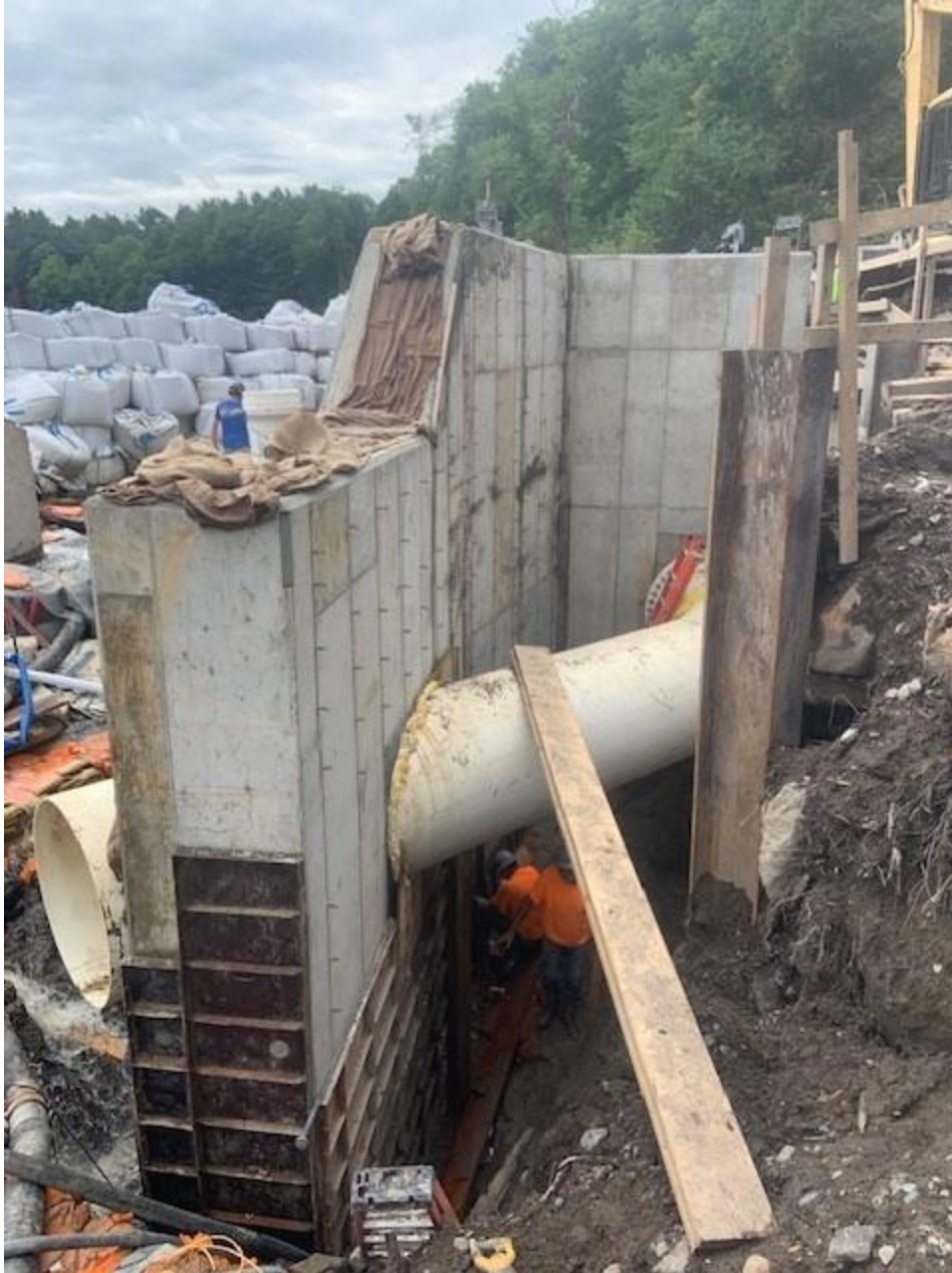
West-side abutment after concrete placement
