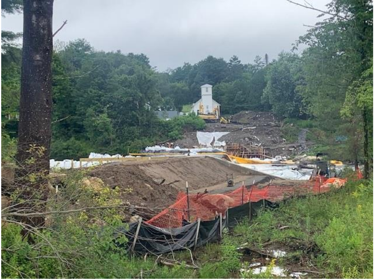
Installation of east-side embankment dam core material
