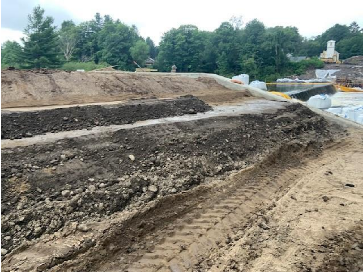
Installation of east-side embankment dam filter sand and gravel.
