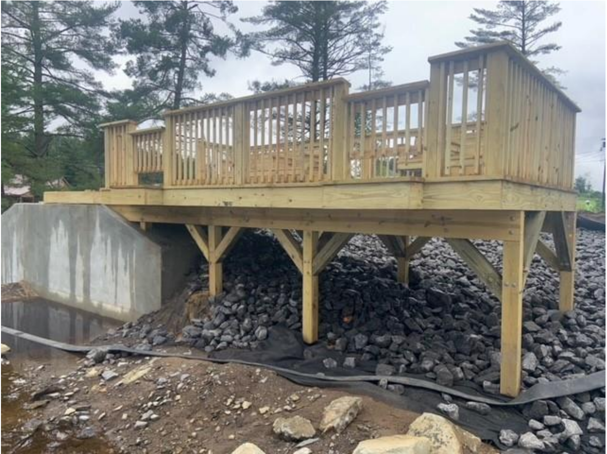
Accessible Fishing Platform nearly completed
