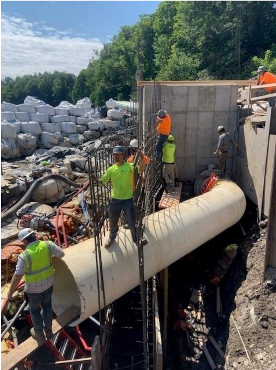
Installation of the outlet pipe and west-side abutment
