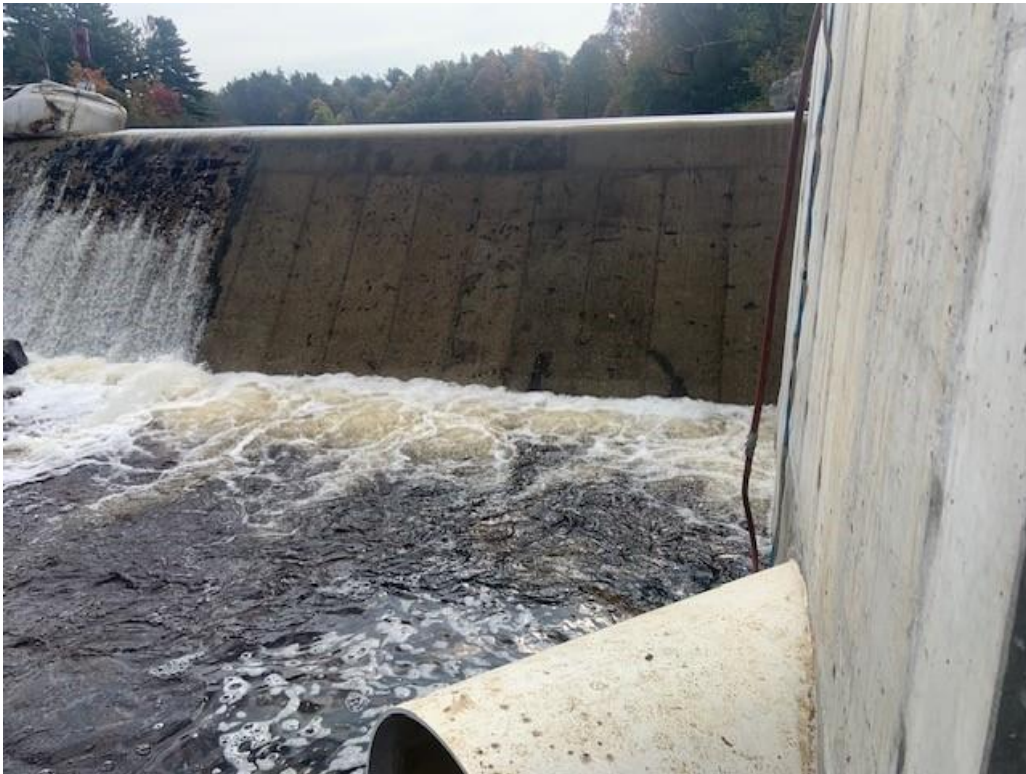
New Spillway Section
