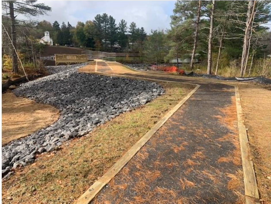
Earth Embankment Dam
